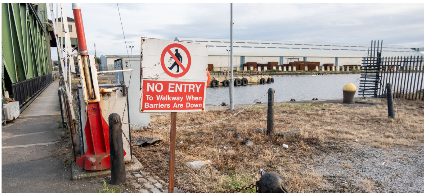
West Float Industrial Estate, Birkenhead
